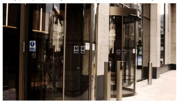
Curved sliding door systems are available in several different variations from complete circular doors containing a pair of external and a pair of internal doors supported by a glazed drum to creating an entrance vestibule to single door suites to follow the curve of a façade to maintain an uninterrupted aesthetic.
