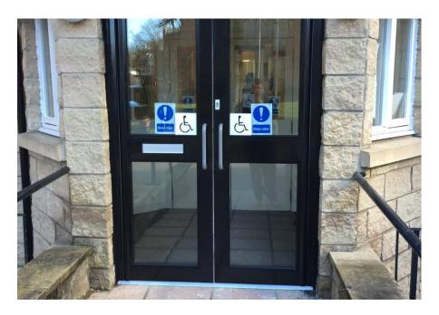
Debridge Doctor's surgery in Bearsden in Scotland. This is a DFA 127 FULL POWER DOOR. As this door has a programmable micro-processor the speed of opening and closing can be adjusted.
