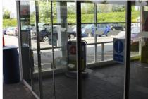
This is an installation of the **record uk** telescopic TSA20 at the Tesco store in Rugby. The store required an entrance capable of allowing the safe passage of large numbers of people at one time, and at the same time not leave the entrance open to the elements for unduly long periods. This was achieved by the installation of automatic folding doors at both sides of the wide entrance, thus allowing maximum access while mimimising rapid ingress of cold air and dicomfort for customers and staff.
