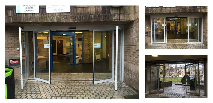
This record Total Opening System (TOS) was installed at the entrance to the Geographical and Earth Sciences department at Glasgow Caledonian University. The TOS system allows these sliding doors to be released to provide the widest possible escape route in the event of an emergency.
